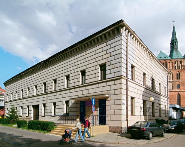
Knight Academy rebuilt following the ravages of war, today it hosts a sports hall.
